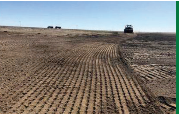
After all the rig mats and temporary roads were dismantled, the impacted areas were harrowed and seeded with an approved seed mix.
