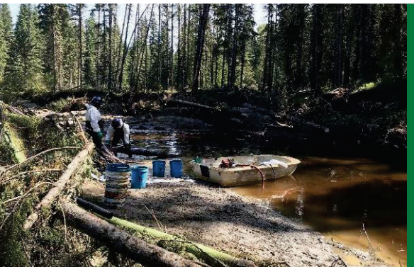
The SCAT crew utilizing portable low flow pumps to wash the impacts from the fallen woody debris within the release area.
