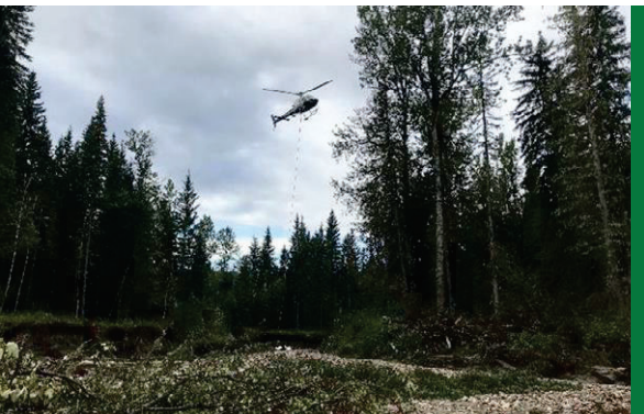
Using a helicopter to longline impacted material from the creek to the staging area in preparation for disposal.
